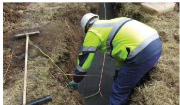
possible the copper conductor must be coiled back from the furthest point and run back along trench towards the DSLAM plinth hole, ensuring the coiled back section does not touch the surrounding earth and is covered by conductive concrete material.
