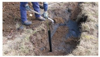
Please note: If the earth free from stones from the excavation is of poor quality or not available due to the particular local ground conditions (e.g hard rock or type 1 only material) then Contractor MUST consult with local Openreach Contracts Manager regards sourcing suitable alternative soft soil (e.g via local purchase) — this initial layer of soil must be hand tampered before subsequent layers of backfill material are applied.
