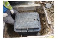
Every system can be supplied with a standard Ductile Iron Cover or Concrete- Filled Cover.
