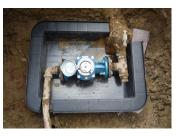
Sections can be cut on site to allow pipes to run through the chamber.
