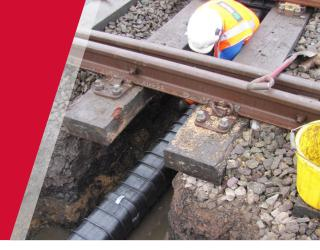
Cubis' UTX system is a Network Rail-approved method of building under track crossings that are faster, safer and cheaper to construct.
