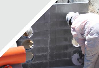
Ducts can be drilled a minimum of 50mm from the inside edge of the chamber.
