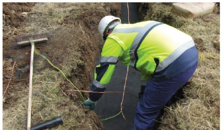
Ensure the copper electrode is run for the full length of the duct trench (ideally for 2m). If this is not possible the copper conductor must be coiled back from the furthest point and run back along trench towards the DSLAM plinth hole, ensuring the coiled back section does not touch the surrounding earth and is covered by conductive concrete material.
