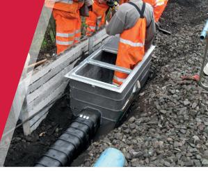
In addition, the tried and tested design of the STAKKAbox<sup>™</sup> means that when installed, the unit will provide years of service for Network Rail. The STAKKAbox<sup>™</sup> is not affected by diesel, ground acids, alkalines or frost – all known killers of concrete. As a structural unit it will support loadings imparted from vehicles and passing trains.
